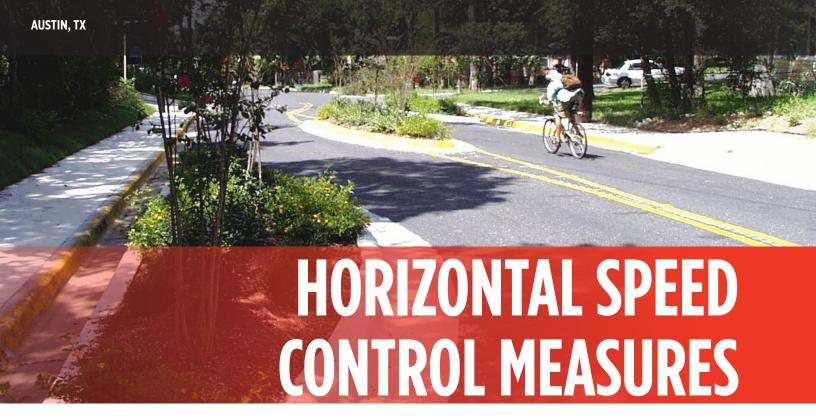
Horizontal speed controls reduce traffic speeds and reinforce safe, pedestrianfriendly streets by breaking up the linear path of vehicles through horizontal shifts. By forcing drivers around horizontal curves and blocking long views of the road ahead, vehicle speeds can be reduced on neighborhood streets. Horizontal deflections include chicanes, neck-downs/chokers, and center islands. Mini-traffic circles are also a form of horizontal speed control.
