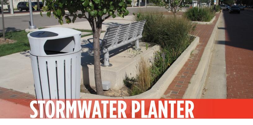
A stormwater planter is a vegetated green infrastructure practice relying on specified soils and vegetation to treat and absorb stormwater. It is different from other vegetated best management practices as it typically has concrete vertical side walls allowing it to be incorporated into congested street corridors or attached to the perimeter of a building.
